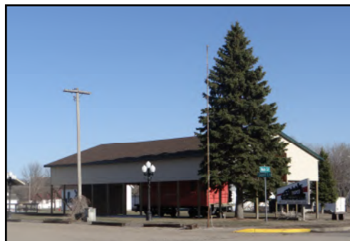
Caboose building and restrooms
